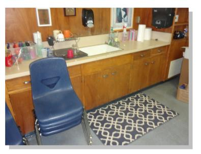
Photo -2 The typical sinks in the classrooms have not been upgraded to current accessibility standards
