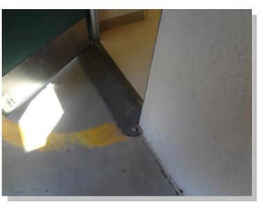
Photo -4 Thresholds are not current with accessibility standards.
